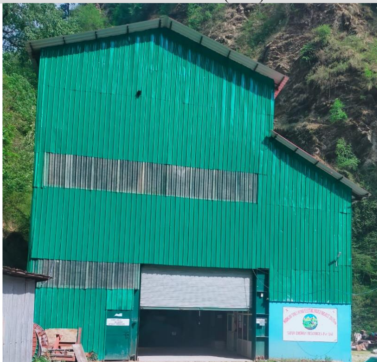
3.5 MW Small Scale Hydro Power Project
